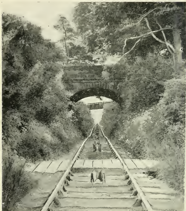
Swannington Incline, on the old Leicester and Swannington Railway
